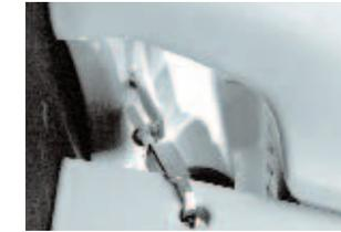
The installation bracket developed by LAUFEN allows the front panel to be removed quickly for thorough cleaning.
